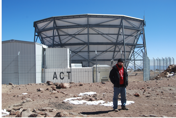
Figure 6.1: The Atacama Cosmology telescope. The telescope is located inside the large, visible ground screen, which mitigates pickup of systematic noise from the surrounding terrain from entering the telescope sidelobes. The structures in the foreground contain equipment and facilities. Author in the foreground.
